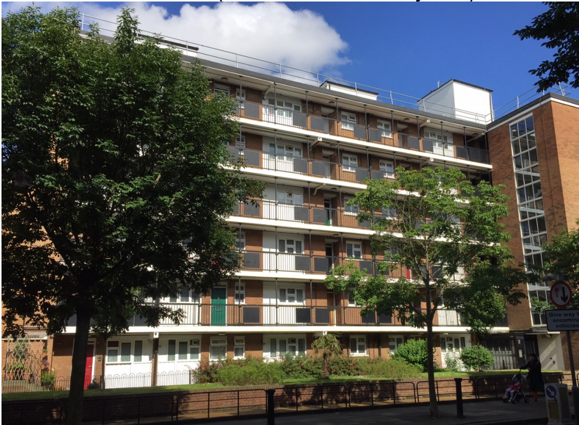
Wexford House (Eastwards View from Sidney Street)
